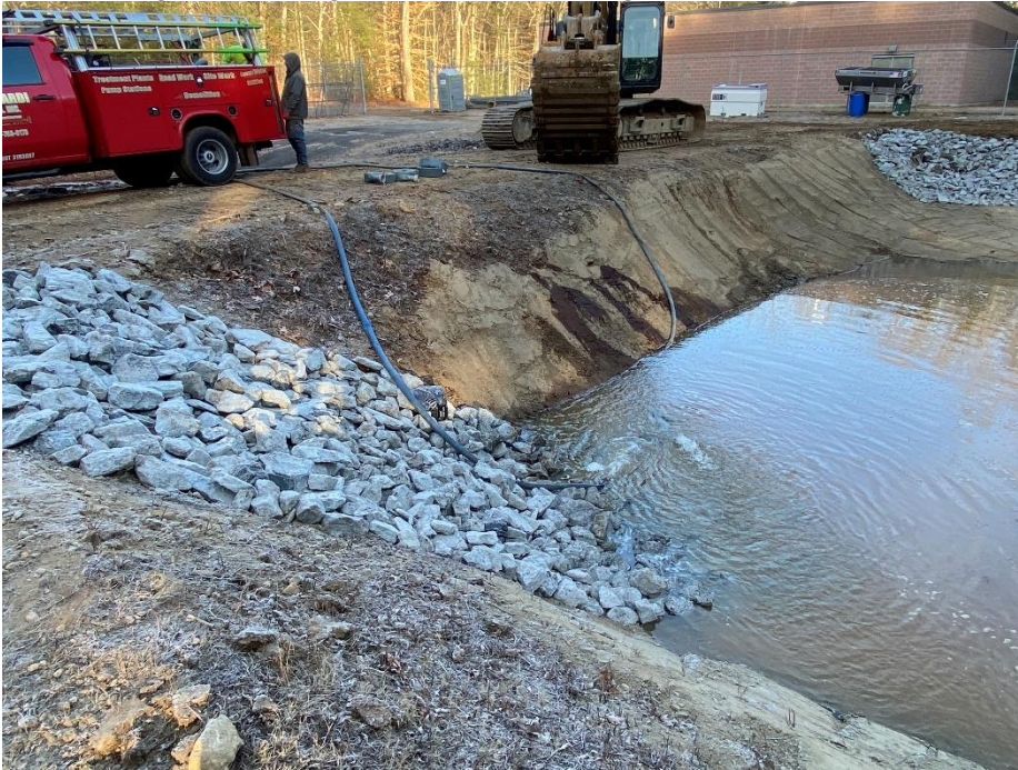
Photo – Lagoon 2 being dewatered into Lagoon 1
