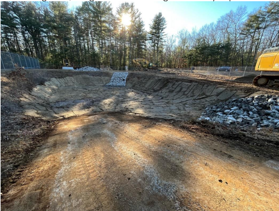
Photo – Lagoon 1, sludge is removed & lagoon is ready to put back in service
