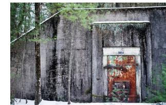
**Bunkers**—30 soil-covered ammunition bunkers (“igloos”) with concrete cores were constructed at the Annex in 1942. War materials were moved on and off railroad cars and stowed in the bunkers, with access through their massive steel doors. Ammunition arriving in Boston was sent by rail for storage in the “igloos”. It was sent back to Boston Harbor by rail when needed for the war effort. Vestiges of old rail beds are still seen in the refuge. Bunkers measure 81x26x12 ft.
