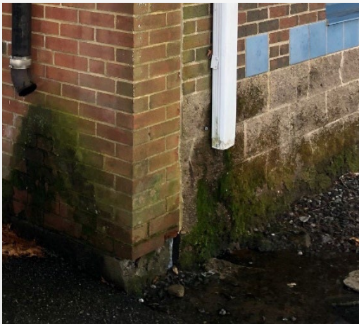
Deteriorating/ Cracking Masonry
