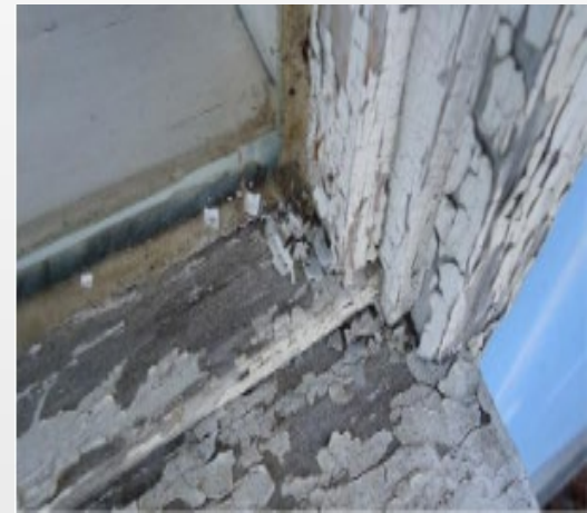
Deteriorating Window Framing
