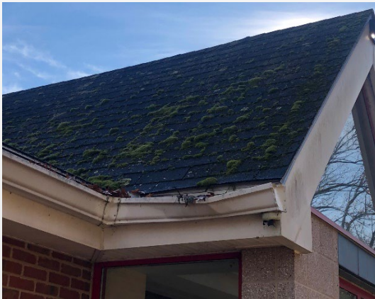
Deteriorating Roof/Damaged Gutters
