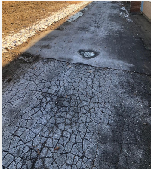
Deteriorating Paving at Play Areas
