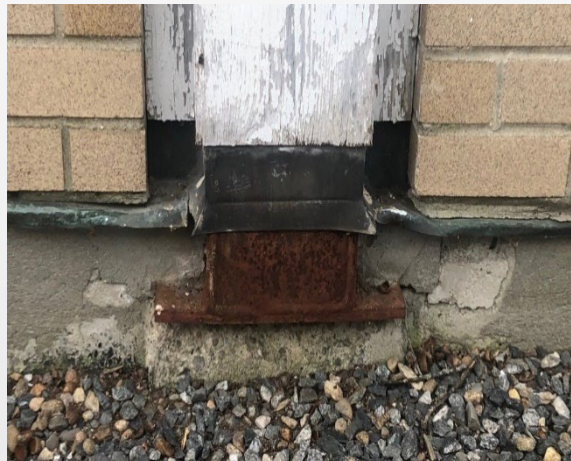
Exposed Steel Columns
