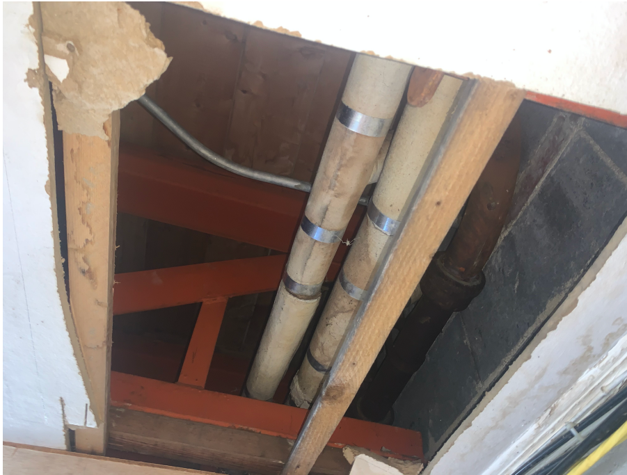
Figure 1: Pipe insulation is asbestos-containing.
